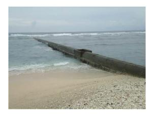
Figure 5. Sewage Ocean Outfall Structure
