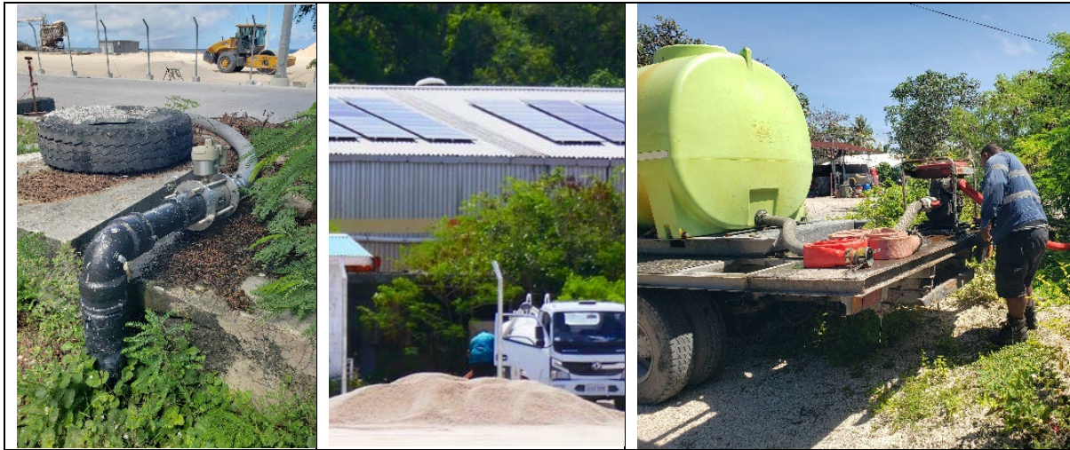
Figure 12-2 RO intake pipe near port (left), water truck refilling at RO plant (middle) and delivering RO water to household tanks by truck (right). Photo credit: CSIRO, 2024.
