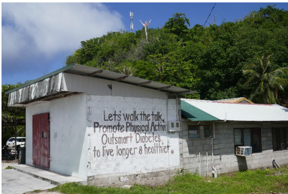
Figure 13-1: Health message on a building. Photo credit: CSIRO, 2024.
