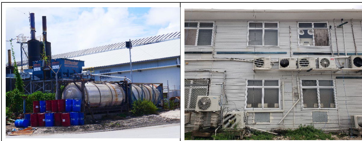
Figure 17-20 Electricity company located adjacent to the port (left). Air conditioning units are common in Nauru (right). Photo credit: CSIRO, 2024.
