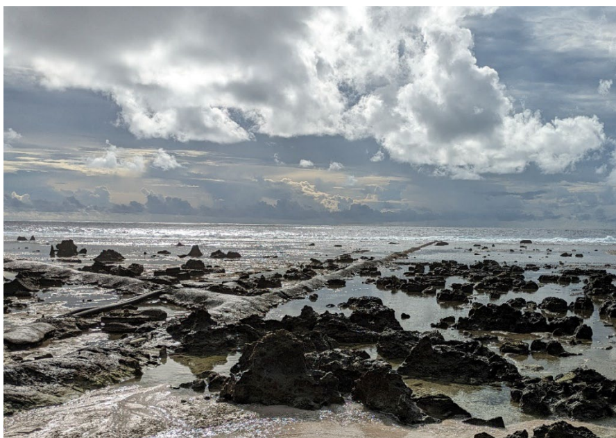
Figure 12-5 Exposed water intake pipes for Meneng RO facility (Photo credit M Sheppard CSIRO, 2024).
