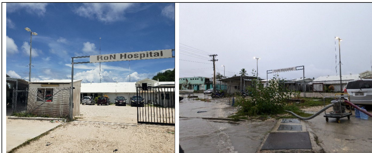
Figure 17-23 Republic of Nauru (RoN) Hospital entrance (left) and in flood after heavy rain (right). Source M Sheppard CSIRO, 2024.
