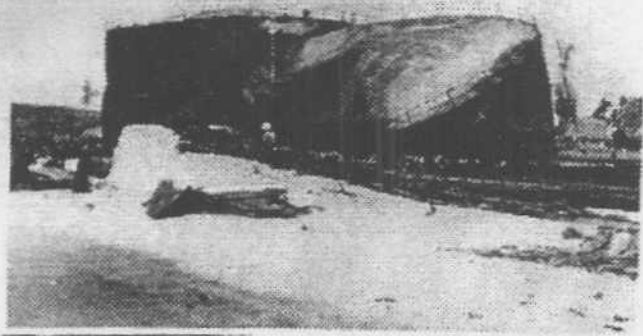
Likewise, the oil drums set afire by the German raider still lay bent and buckled in September 1945. The German attack lasted one hour and 18 minutes, during which 126 5.9-inch, 360 3.7cm and 719 2cm rounds were fired causing extensive damage and stopping all phosphate operations for ten full weeks.
