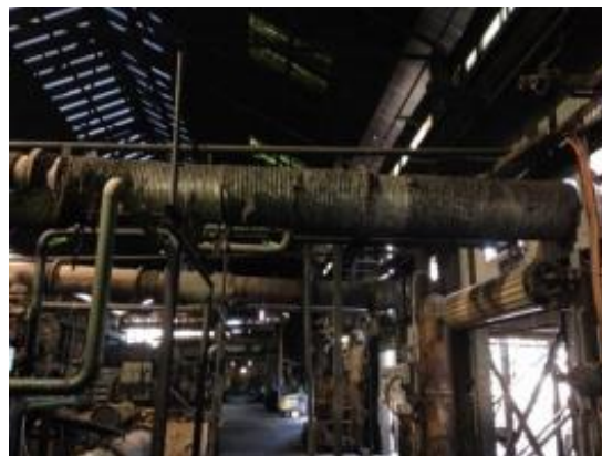
Photo 81 – Fibreglass Rope Lagging
