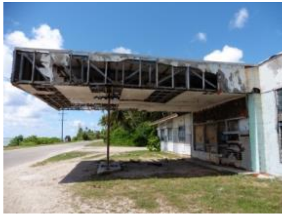
Photo 70 - Abandoned Petrol Station
