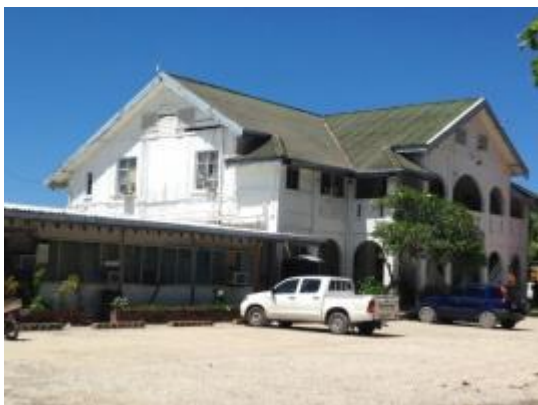
Photo 40 - Central Office Building
