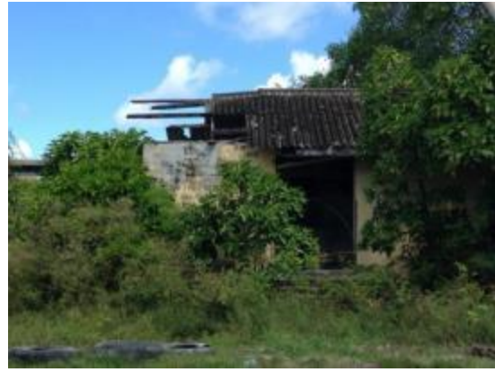
Photo 69 - Derelict Building Aiwo
