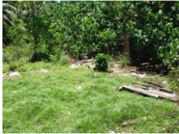
Photo 6 – Asbestos on Ground Behind House
