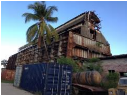
Photo 44 - Old Phosphate Storage Bin by Hotel
