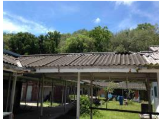
Photo 16 – Hospital Parapet Roof
