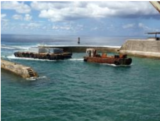
Photo 84 - Barge and Raft
