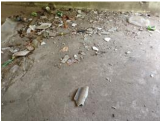
Photo 13 – Asbestos Debris around House
