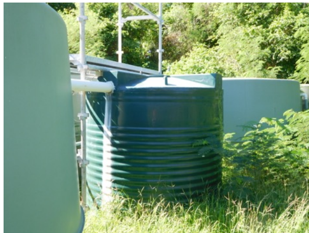
Figure 22. A replacement tank has been installed at the plant
