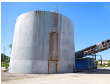
Figure 13. Tank 'B13' remaining – tank 'B10' demolished (by May 2017)
