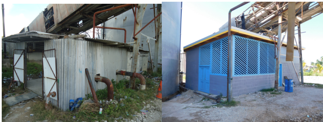
Figure 15. Pump Station Building Before (2015) and After Upgrade (May 2017)
