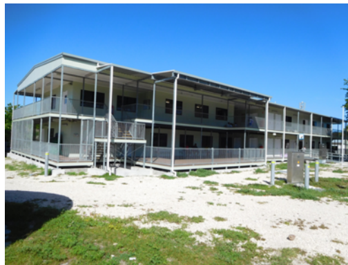
Figure 19. New School Building At Nauru Primary School
