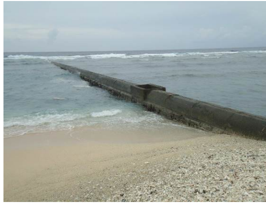
Figure 5. Sewage Ocean Outfall Structure
