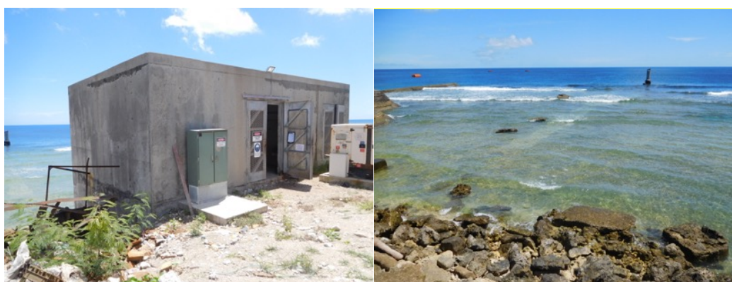
Figure 8. Existing Seawater Intake Structure and Inlet Pipeline to Marker at Edge of Reef
