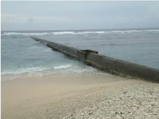
**Figure 5. Sewage Ocean Outfall Structure**
