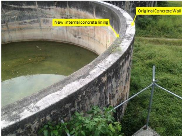
**Figure 30. Past Remedial Works at Command Ridge Tanks**
