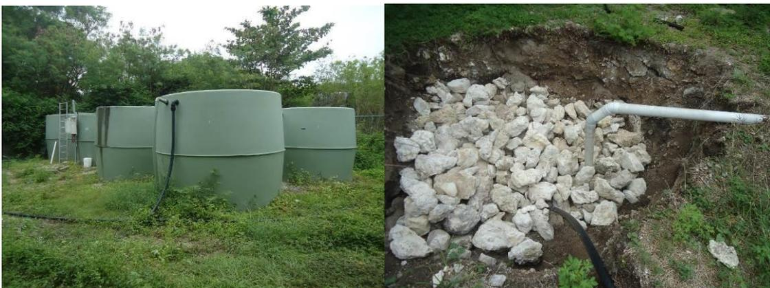
**Figure 6. Sewage treatment Plant at Nauru Primary School with Effluent Dispersal Pit**
