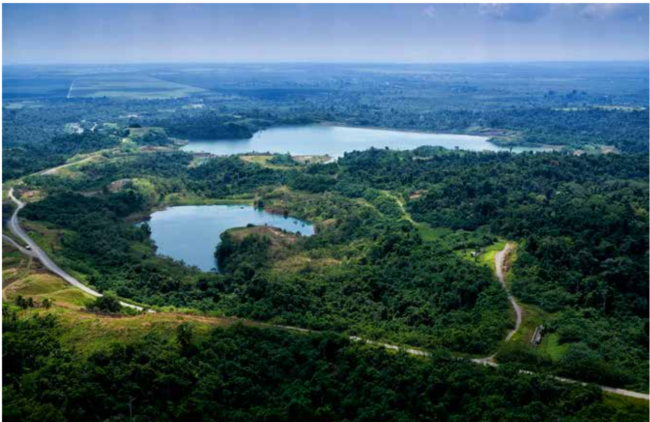
Gold Ridge Mine tailings dam, Guadalcanal, Solomon Islands. © Stuart Chape
