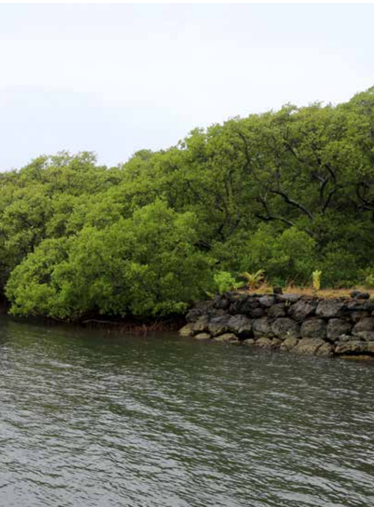
Traditional method: land reclamation integrating natural coastal protection, Yap, FSM. Photo: Greg Barbara
