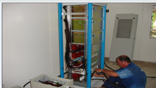
INSTALLATION OF CONTROLS
